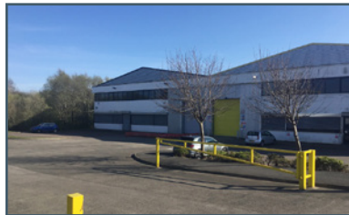
East Shawhead Industrial Estate, Coatbridge Client: Dennis Rye Ltd Size: 7,838 - 10,758 sq. ft.
